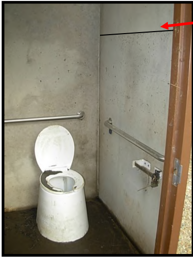
Left: High water level at east pit toilet in Alcock Park Below: Tree damage east side Alcock Park
